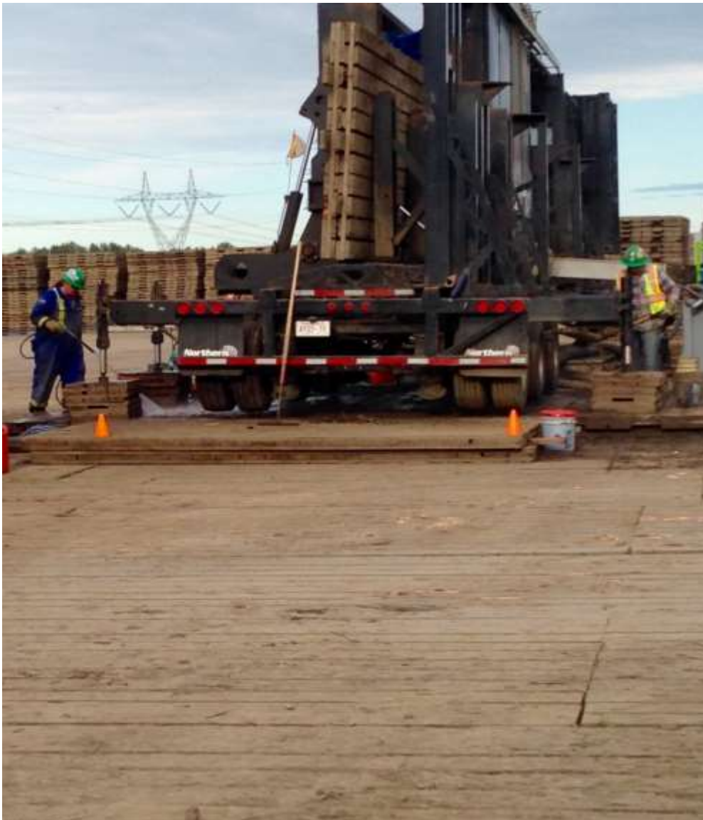
MATS BEING PLACED ON THE LAND
