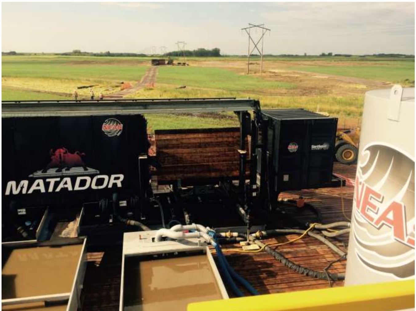
MATADOR MAT WASHING STATION IN ACTION
